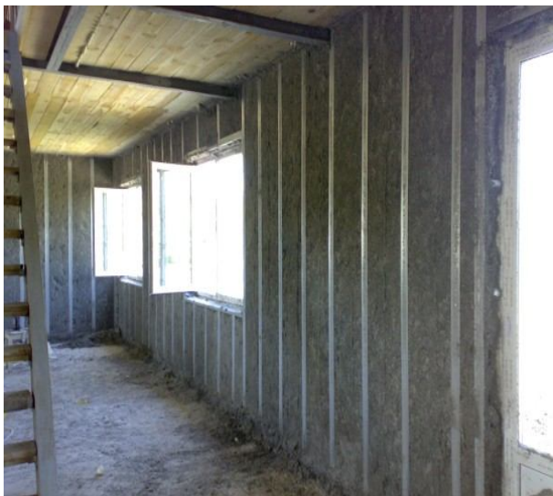
Fig. 7. Additional walls insulation of already erected building
