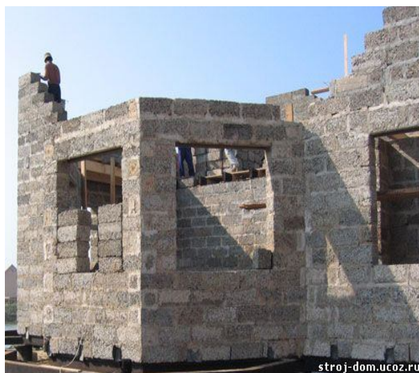
Fig. 5. General purpose building made of sawdust-cemented blocks
